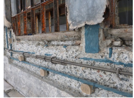
Window-sill mock-up showing corrosion inhibitor and cathodic protection.
