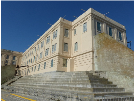
Historic cellhouse repairs completed
