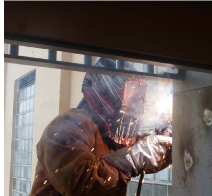
Recreational yard door installation
