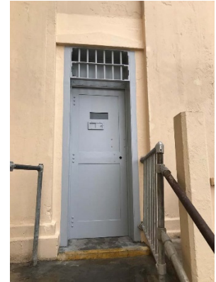
Recreational yard door completed
