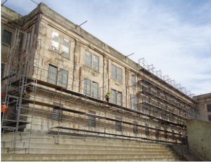
Cellhouse exterior being readied for repair.
