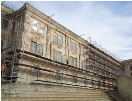
Cellhouse exterior being readied for repair.
