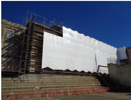
Shrink wrapping provides a visual barrier so that work does not disturb the island's birds.
